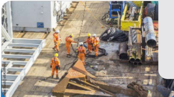
Buoy Maintenance Construction Support Activities
